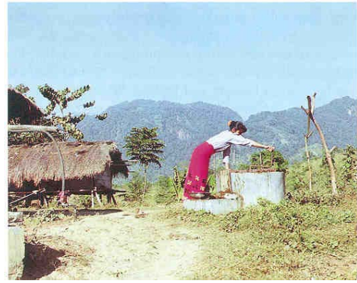
Deenbandhu Plant in use in Arunachal Pradesh Source: Ministry of Non-conventional Energy Sources < http://mnes.nic.in/frame.htm?majorprog.htm >
